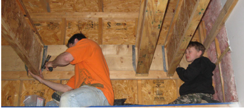
Tim and Luke Zello nailing the floor joists.
